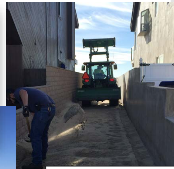
Clearing of easements
